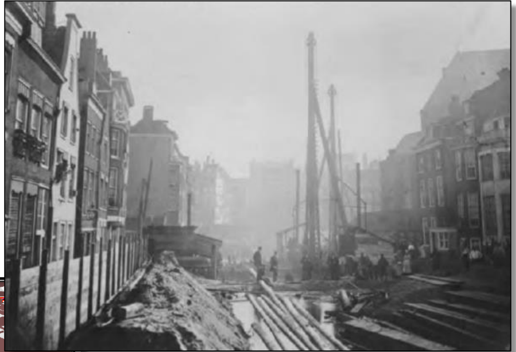
Example of wooden pile (1879)
